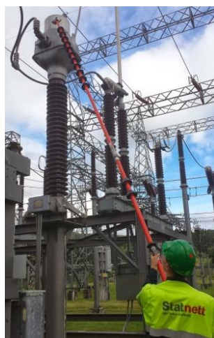
Use of camera with insulation rod.
