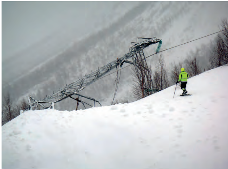
AutoDig automatically identifies and reports operational interruptions in the power grid.
